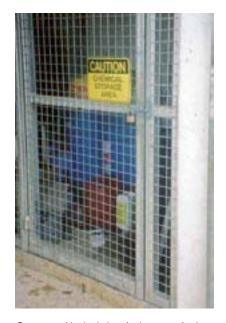
Secure and locked chemical storage in the dairy with concrete floor and bunding to contain spills.
