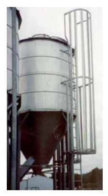
Ladder cage that incorporates a locked restricted access panel.
