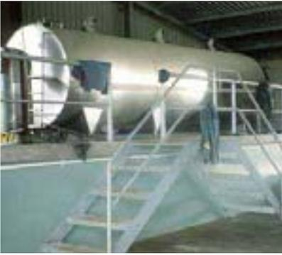
*Well constructed steps and handrails.*
